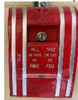
Two Stage Fire Alarm Manual Pull Station
